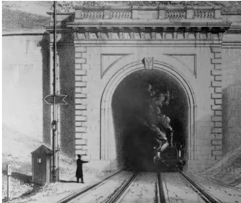
Western entrance to Box Tunnel, Corsham, Wiltshire - built by Isambard Kingdom Brunel and opened in 1841
